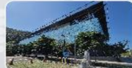
DC Yilan station
