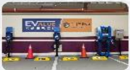
DC Tucheng station
