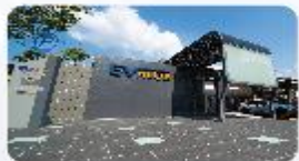
DC Neihu station
